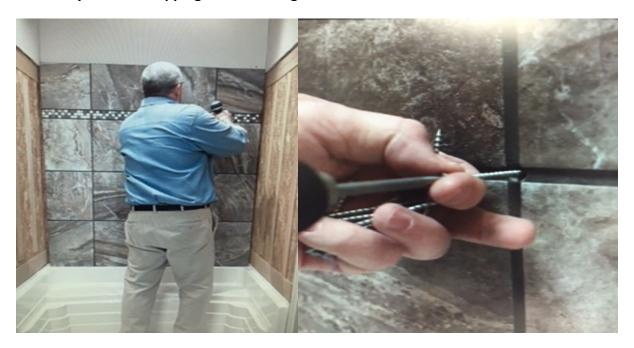
In the kits with multiple wall sections install the wall panels in the numbers sequence as marked on the panels.
