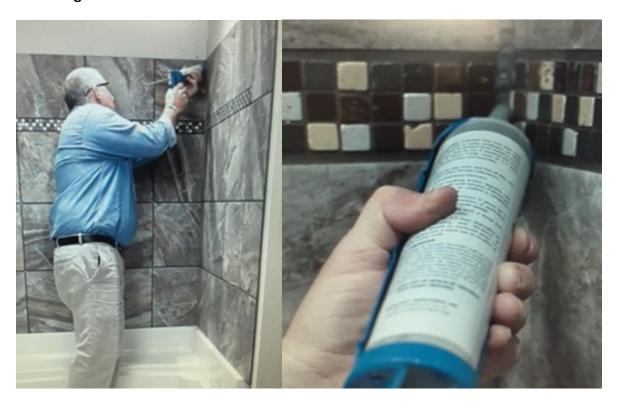
Next: Install pre mixed grout(supplied) to screw holes and open grout lines (where two panel meet and bullnose). All grout used in the wall panels and the pre mixed supplied grout is pre sealed and does not require any sealing after the install is complete.
