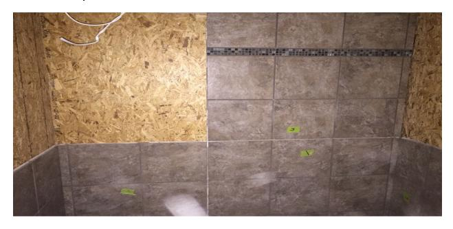
Once the back wall panel(s) has been installed, install either of the side panels. If the panel is on the wall that has the shower diverter lever or knobs, measure and cut these prior to installing this panel.
