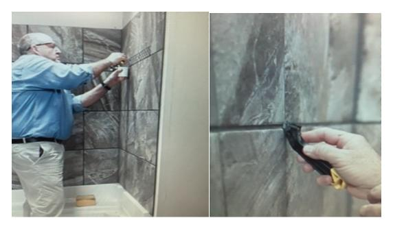
Immediately after grouting screw holes, bullnose and open grout lines sponge these areas with a damp sponge. Wipe lightly over the other creating a feathered application to ensure that the grout dries to match the existing grout lines.
