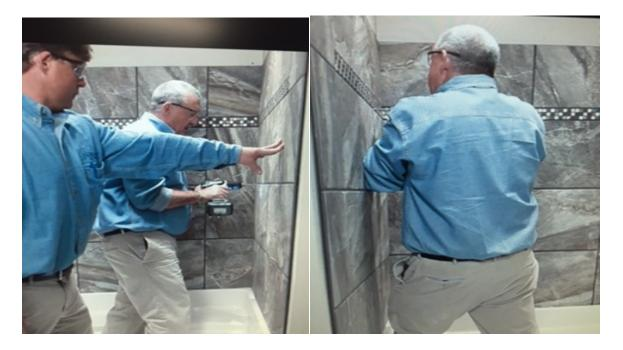
NOTE: When applying a wall panel that is joining another panel, be sure grout lines are lined up properly and adjoining panel or side panel is pushed as tightly as possible to adjoining wall before securing to the wall. This will insure minimal grouting or caulking.
