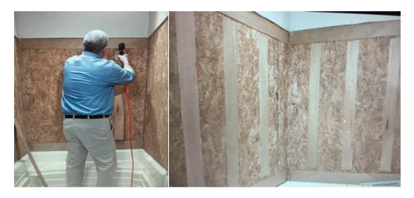
The back wall is always installed first. If the back wall is 2 pieces install the bottom section first. This wall may be numbered as 1.
