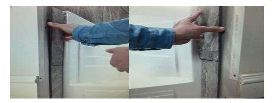
Be sure to use ¼" spacers if multiple pieces are installed to ensure uniform grout lines with wall panel grout lines.
