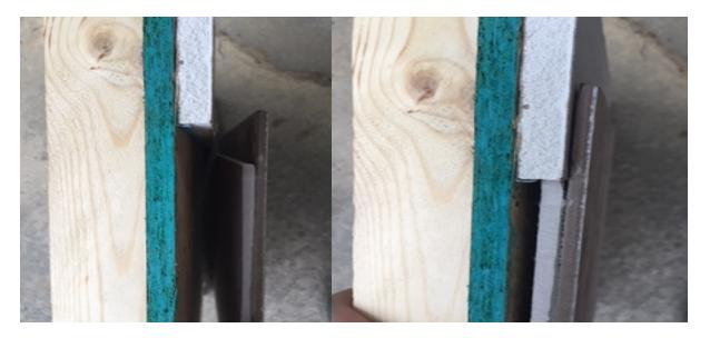
If  $\frac{1}{2}$ " or  $\frac{3}{8}$ " Sheetrock or VOG in used furring strips are not required. If  $\frac{1}{2}$ " sheetrock or VOG is used then  $\frac{1}{8}$ " or  $\frac{1}{4}$ " strips are need to be installed prior to the wall panel installation to ensure that the backer will be against a solid wall without space between the backer and the OSB.
